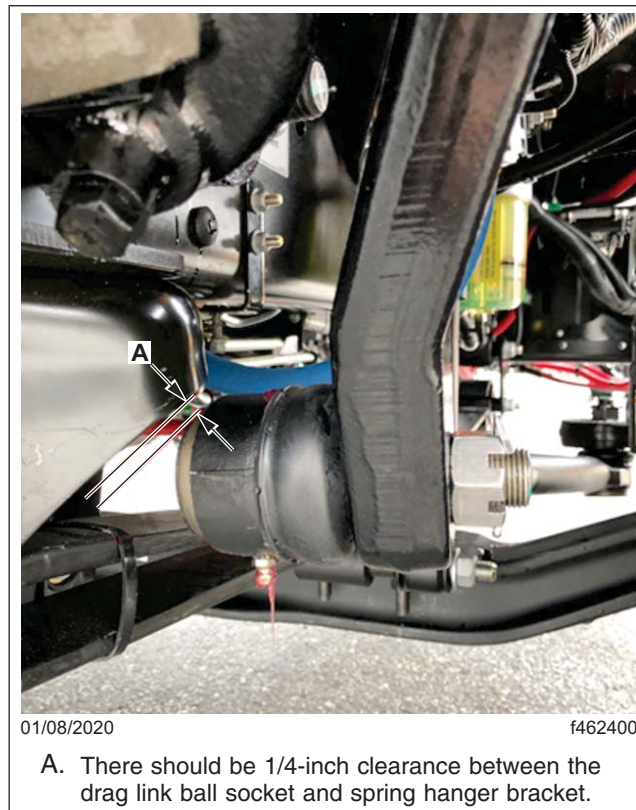
Fig. 1, Inspecting for Proper Clearance
