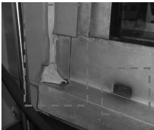
Figure 6 and 7: Unacceptable - Cracked and dry old caulk and drain holes needing repairing
