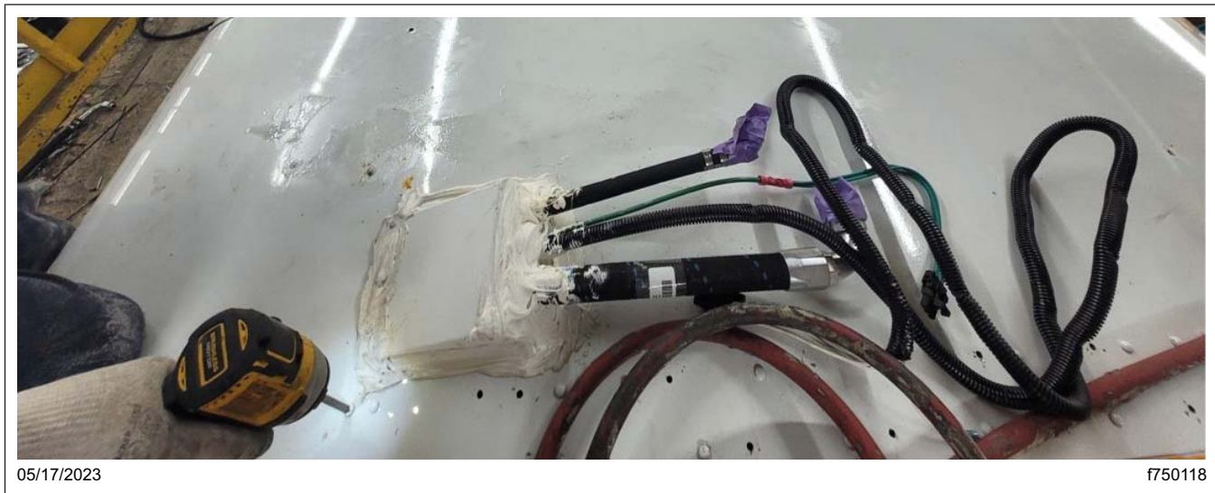
Fig. 14, Installing the Screws along the Joint
